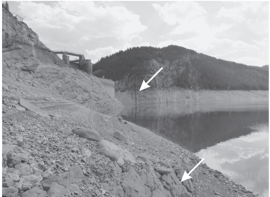
Figure 8. Gibson Dam (left center) with limestone/dolostone dipping west (right) at 83^\circ as seen across the Gibson Reservoir (center). Sandstone bed near the contact with the limestone/dolostone dipping west at 79^\circ .
