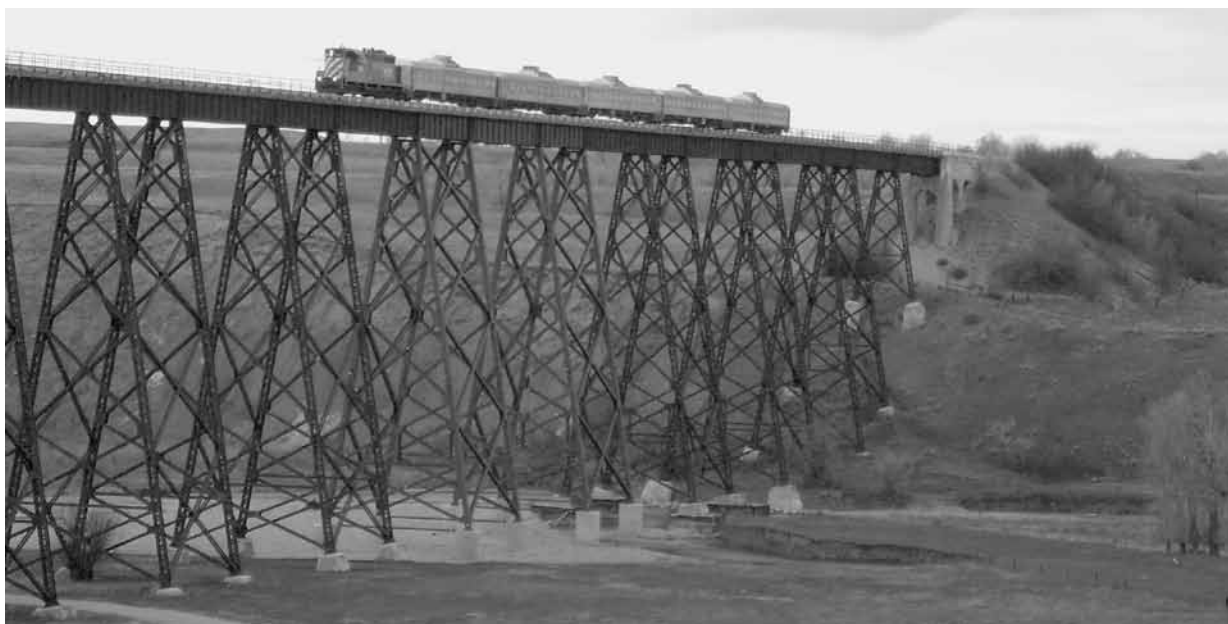
Figure 10. The first revenue train following repair of the viaduct was the Charlie Russell Chew Choo dinner train on November 21, 2014. Grain trains still had to wait for repair of the Ross Fork Bridge. Note the new piers supporting bents directly under the train. Photograph courtesy Central Montana Rail.
