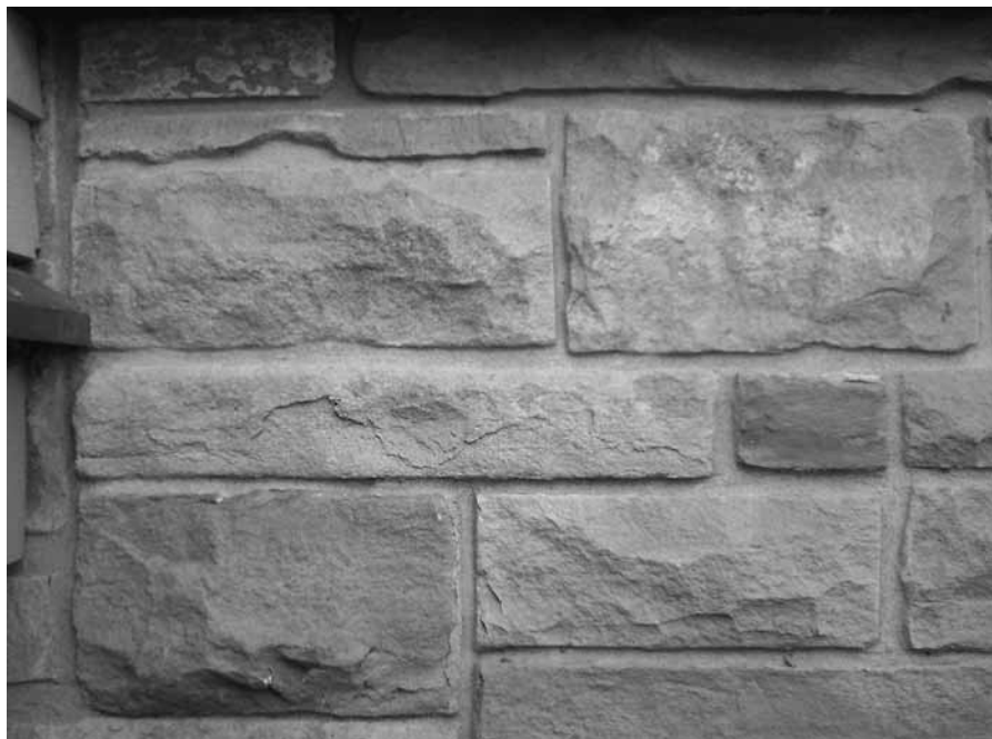
Figure 2. This 30-year-old reinforced stone foundation was built with upper Kootenai sandstone quarried 135 years ago, refaced, and reused. While the reinforced concrete piers and grade beams it sits on have an unconfined compressive strength of 5,000 psi (34 MPa), the sandstone averages 11,000 psi (75 MPa). The primary stone is a medium-bedded arkosic sandstone (immature, fine-grained to medium-grained subarkose) with minor iron cement; some of the stone is argillaceous (sublitharenite) but it still exhibits a strength of at least 7,000 psi (48 MPa).
