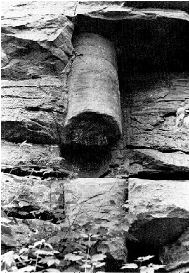
Figure 5. This shows one of the pillars at Hughes' farm. A section has broken out. Marks adjacent to the pillar wall, in the rock adjacent to the pillar, can be seen at the left.
