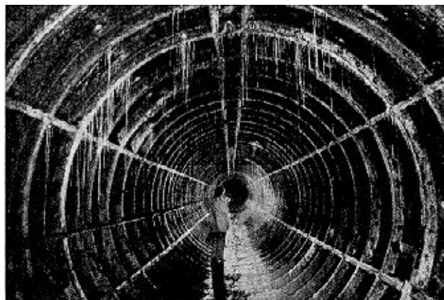
This picture, showing stalactites in an abandoned tunnel, is by the Times of London, as cited, and is used here by permission.
