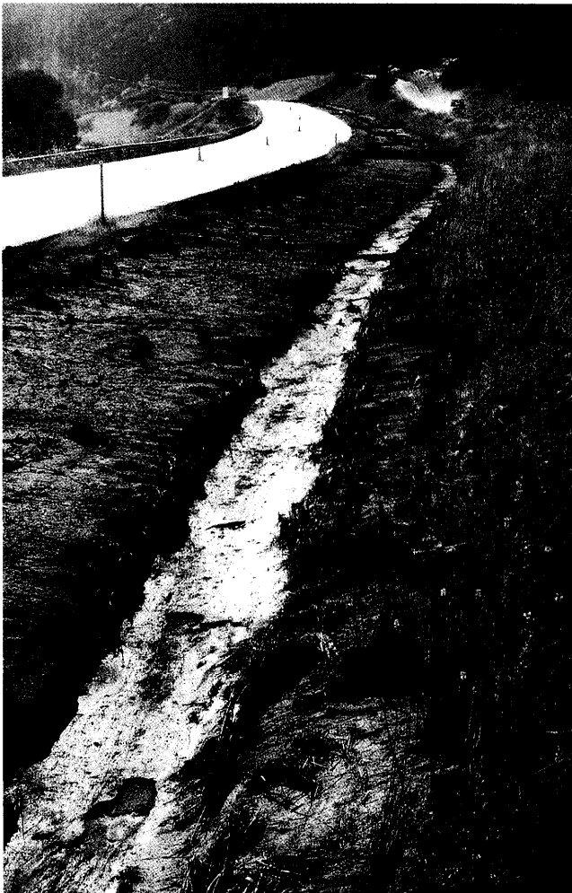
Figure 19. Much of the mud component diverted to the highway gutters, as shown here, and traveled farther across a lesser gradient than the boulder flow that crossed the Interstate on its way to the Colorado River.
