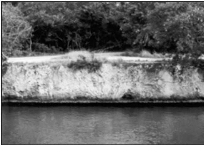
Figure 7. A section of the eastern sidewall along the Marvin D. Adams Waterway showing chunks of limestone which was formally a coral reef environment. The wall extends eight feet above the water.
