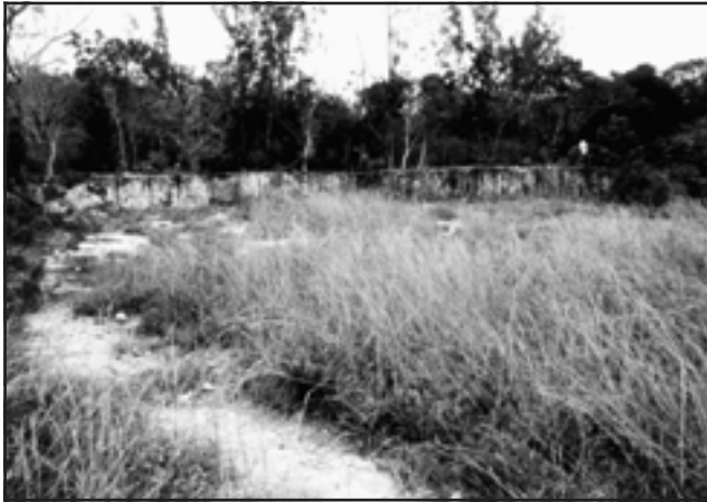
Figure 9. The eastern side of the Windley Key quarry where blocks of limestone were taken for the construction of the railroad which connected Miami to Key West. The sidewalls are from five to seven feet high.
