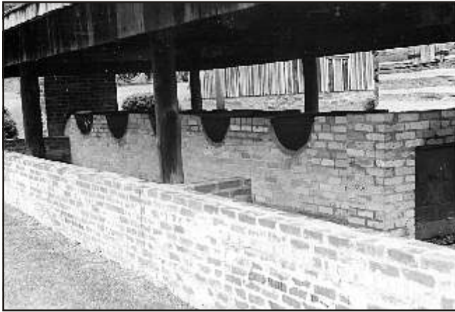
Figure 3. Replica of salt furnaces with kettles in which brine solutions were evaporated, Saltville, Virginia.
