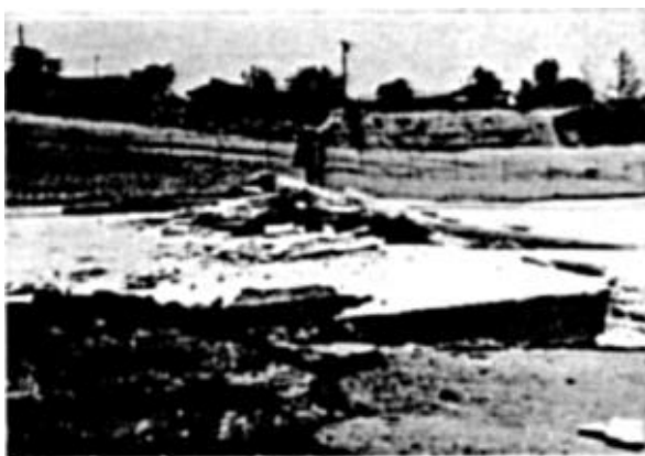
Figure 1. Interstate 210 fault line in concrete: overall view. As the concrete was broken, whole slabs were shoved across other slabs during the earthquake. Barbara Howe is seen in this and other photographs.
