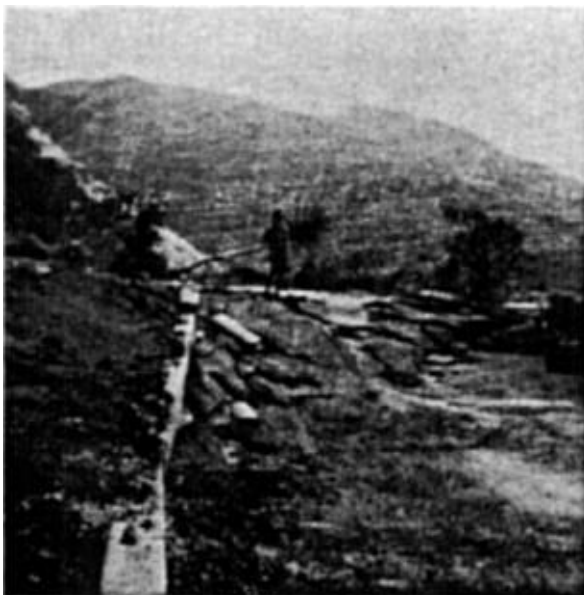
Figure 8. Overall view of twisting and faulting in blacktop of Blue Star Trailer Court, San Fernando, California. The fracturing, slanting, and toppled nature of the blacktop would in itself be evidence of overthrusting.
