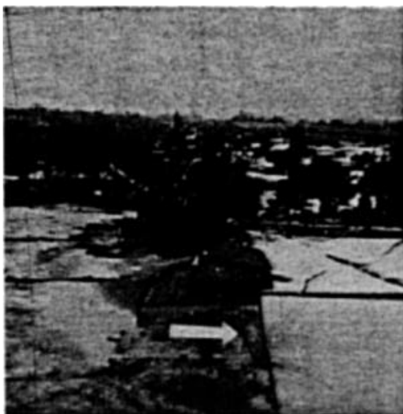
Figure 9. A blacktop, concrete overthrust. Philip Howe is standing on a blacktop slab which was moved some three feet laterally southwestward (direction of superimposed arrow) during the San Fernando earthquake. This is an example of a soft material (asphalt) moving over a harder material (concrete).
