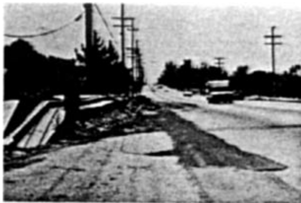
Figure 4. Foothill Boulevard fault escarpment. Here the actual fault line can no longer be seen because of road repair. It is obvious, however, that the sidewalk was elevated several feet in relation to the road bed. This view is toward the southwest, along the fault.
