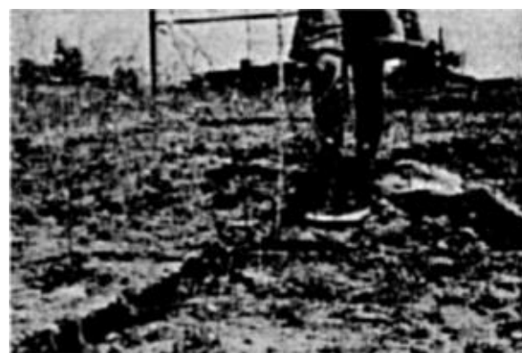
Figure 3. Interstate 210 fault line in clay road bank. North and east of the highway the fault line is visible in the earth fill. There is no evidence of overthrusting in this soft material although the one side of the fissure is now about six inches higher than the other.
