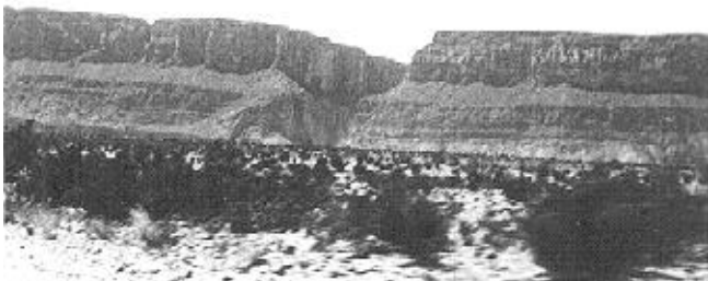
Figure 1. Approach to Santa Elena Canyon showing escarpment face. Sierra Ponce (Mexico) is on left and Mesa de Anguila (U.S.) is on right.
