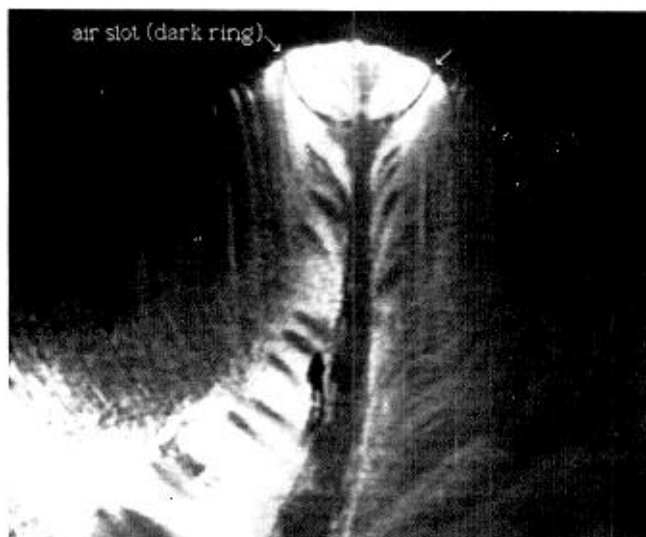
Figure 13. The air slot constructed in the left spillway tunnel of the Glen Canyon Dam is seen as the dark ring at the top of the view. By reducing the speed of sound in the water and somewhat by providing a cushion of air bubbles the new slot now prevents cavitation damage in the spillway by greatly reducing the speed of sound in the water. (From Bureau of Reclamation video)
