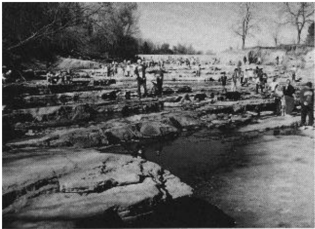
Figure 4. Erosion damage in spillway channel at Coralville Lake. The concrete spillway is visible in the background.
