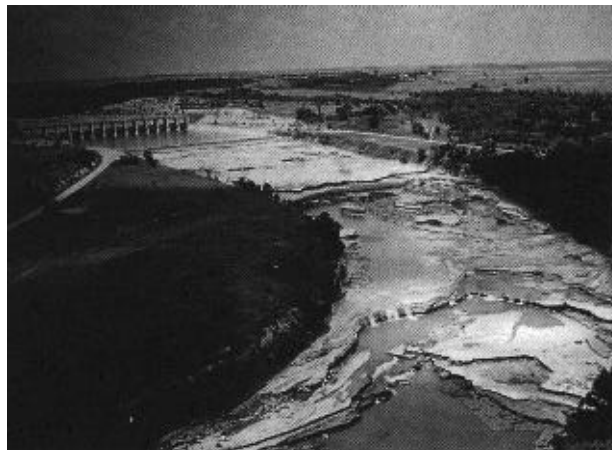
Figure 7. Aerial view of Tuttle Creek Lake spillway area. Photograph by U.S. Army Corps of Engineers.
