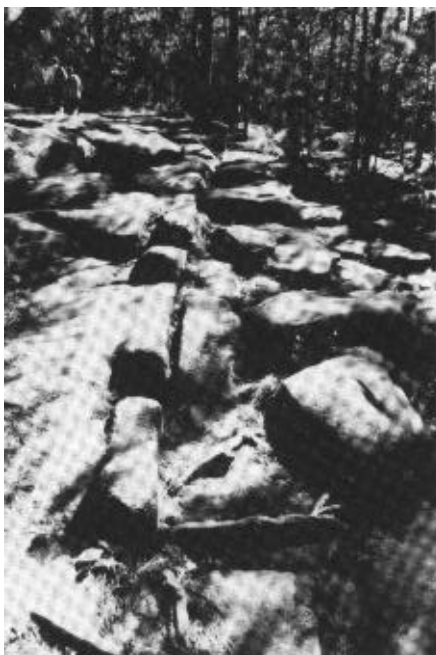
Figure 5. Jointing and weathering of granite has resulted in widening the joints and eroding the jointed rock into blocks.
