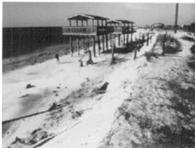
Figure 5. Low tide in January 1994. This photograph shows the more erosive winter cycle of beach erosion. Note considerable landward erosion has occurred since June (compare tree stump positions and beach cliff face). Many more tree stumps are visible during this "winter" cycle. While some sand will be redeposited during the spring and summer cycle, this author does not believe that it will be sufficient enough to stop landward erosion.
