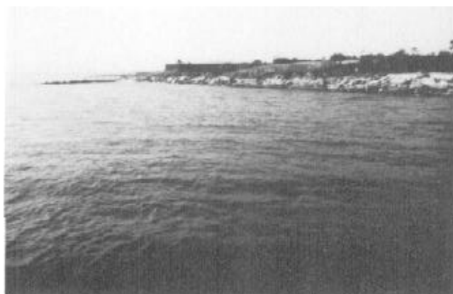
Figure 2. Offshore view of eastern end of Dauphin Island, Alabama. rip-rap has been placed along the shoreline to prevent erosion as sands move from the eastern end of the island towards the west.
