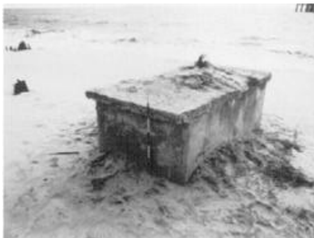
Figure 8. 1000 gallon septic tank. This tank was not exposed during the June 1993 visit to the island. However, the more erosive winter cycle had eroded the sands from around it by January 1994 (a distance of approximately 20 feet). Scale is in 6 inch units.
