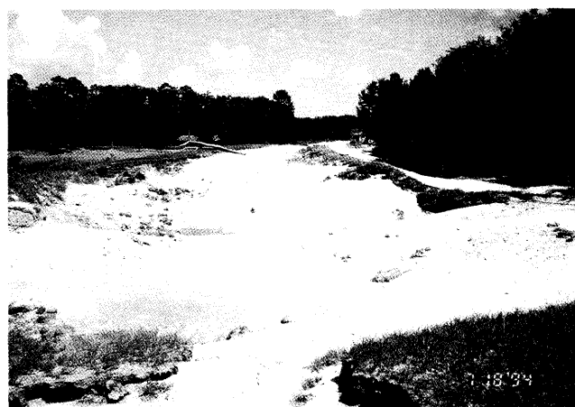
c. Sand deposited by flood waters along interior portion of earthen dike at Lake Worth dam. Photograph furnished by Jack Carson.
