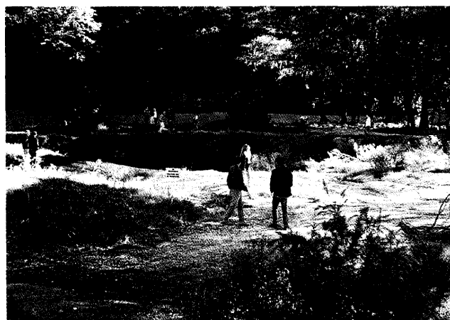
Figure 4. A large, elongated sinkhole located approximately 30 meters west of Kinchafoonee Creek at the northern edge of Albany, Georgia that developed during the flooding of July, 1994. Sinkhole dimensions are length = 44m, width = 21m, depth approximately = 3.1m, volume approximately = 905m 3 . Photograph by Emmett Williams.
