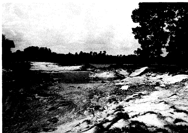
b. Erosional damage of earthen dike at Lake Worth dam. Photograph furnished by Jack Carson.
