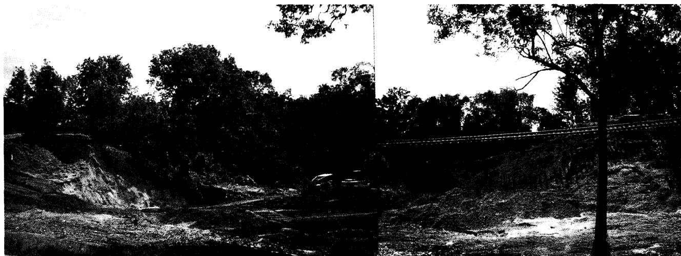
Figure 3. A railroad embankment parallel to state route 49 near Fort Valley, Georgia experienced complete washout during the flooding in July 1994. The photographs were taken nine days after the flood event. Replacement of the embankment had begun. Over one million cubic yards of soil and sediment were removed from this embankment by rapidly moving water in an intermittent stream. When we revisited the site in December, 1995, no water was flowing in the stream. Photographs by Thomas Bruce.
