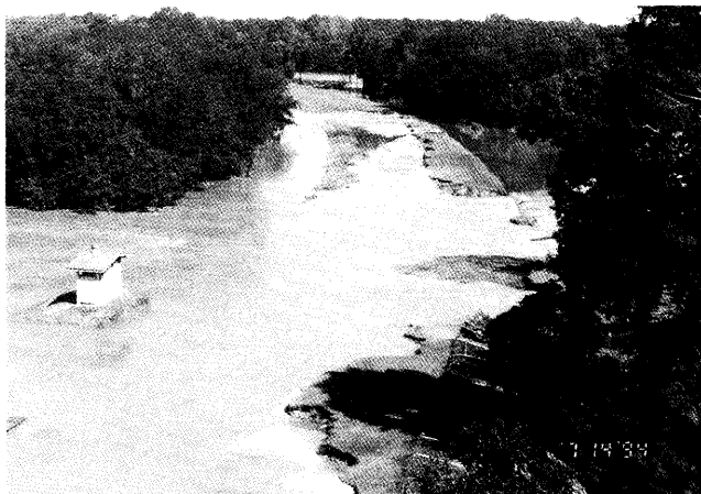
Figure 2 a. Raging flood water overtopping earthen dike at Lake Worth dam at Albany, Georgia. Photograph furnished by Jack Carson.
