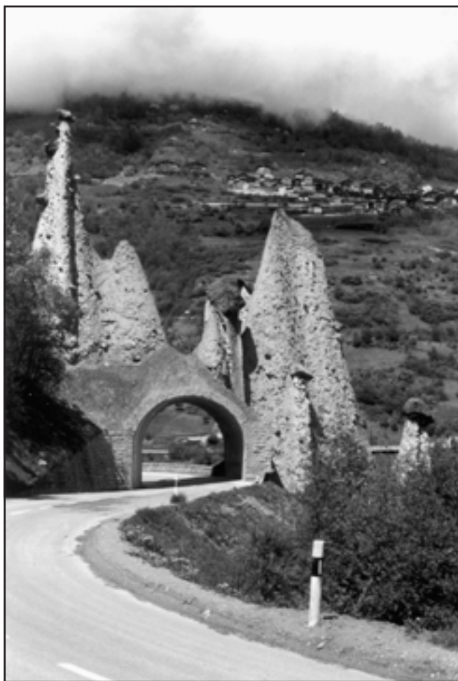
Figure 2. A closeup of the tunnel (opposing side) which has hoodoos above it. Note that the massive column of matrix to the right of the tunnel has lost its cap rock and will now weather in an accelerated manner.
