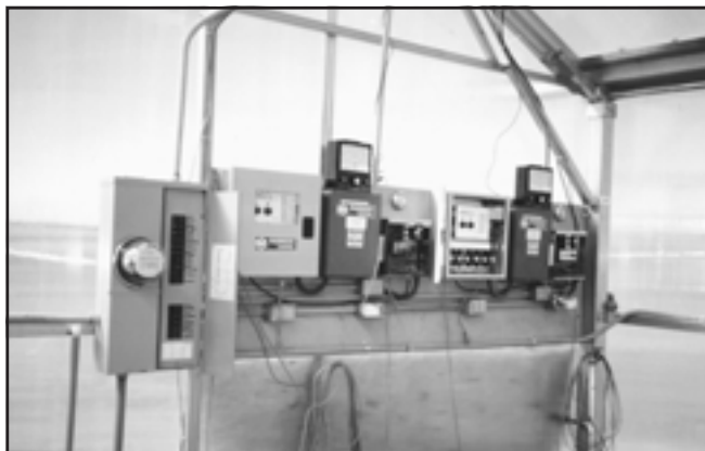
Figure 3. Environmental control units for the research greenhouse.
