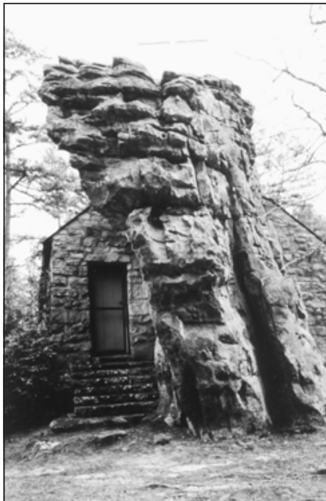
Figure 13. A photograph looking at the front of the church. Note the bedding planes of the sandstone and the slightly offset jointing of the rock spire.
