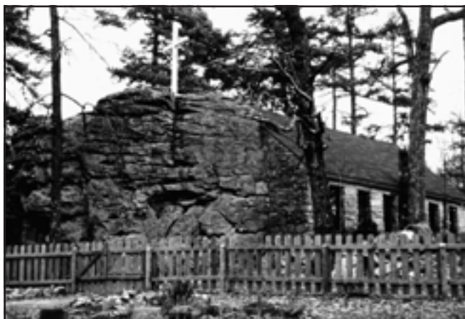
Figure 12. Another photograph showing the opposing side of the pseudo-hoodoo which is incorporated into the front of the church.
