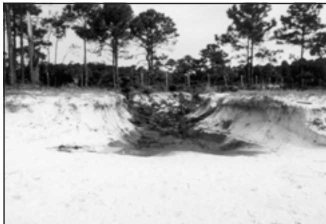
Figure 6. Another drainage channel with steep-sided walls. Note the bifurcation in the flow channels as it moved back into the beach-dune zone. The scale (three feet long in six-inch units) is along the left side of the channel. Brown mud lies along the bottom of the channel.
