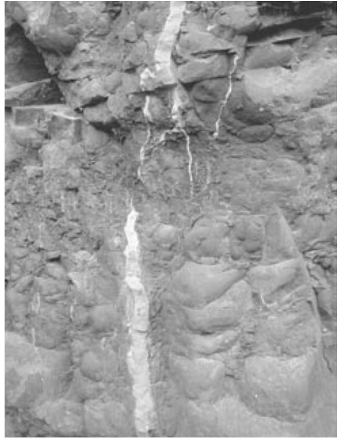
Figure 10. Sand-filled cracks at Dripping Springs, South Rim. Note how the cracks can thin and disappear, and then reappear again. Note how cracks can widen downwards. The U.S. penny, just above the “1” on the largest crack is about 1.9 cm in diameter.
