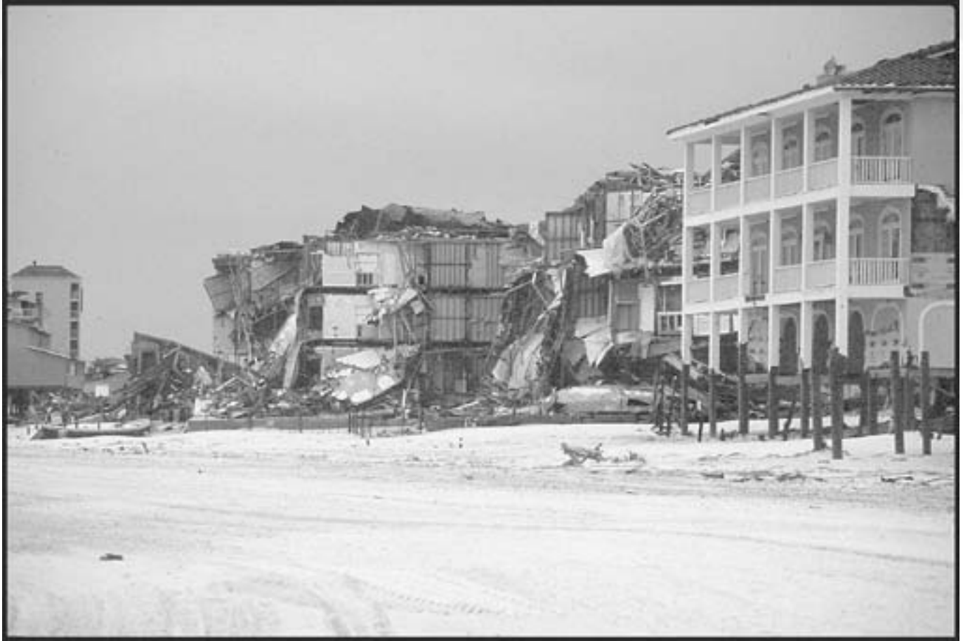
Figure 8. Several condominiums likely constructed on concrete slabs have collapsed due to the severe beach erosion created by the large storm surge generated by Hurricane Ivan. This occurred where sand beneath the slabs was removed during the storm causing structural instability. Note the former sand line along beach house pilings on the right side of the image. Image taken November 13, 2004.
