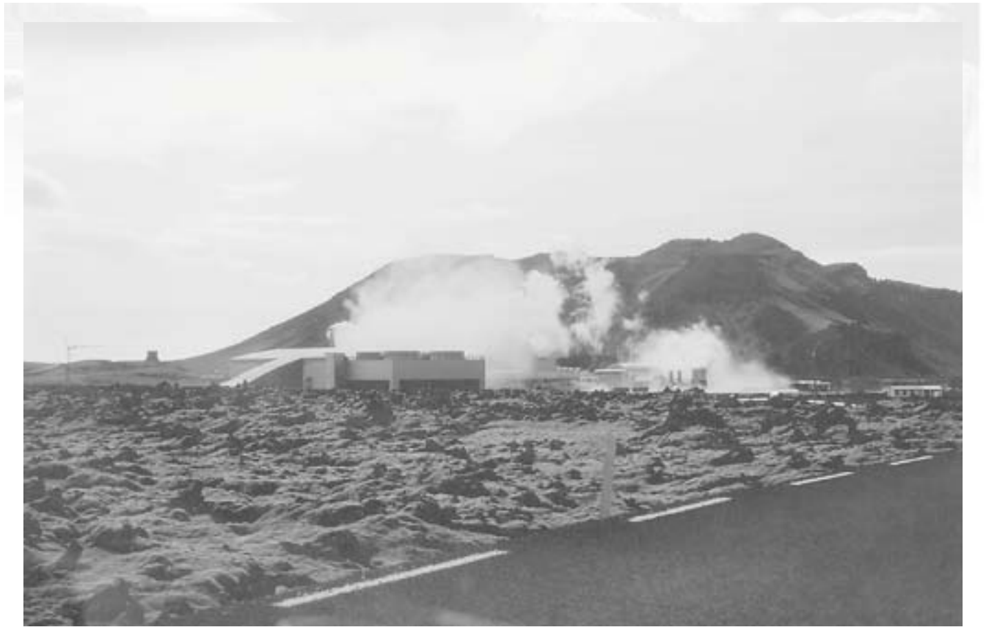
Figure 3. The geothermal power plant responsible for the Blue Lagoon. It is located in a field of tholeiite flows on the Reykjanes Peninsula.
