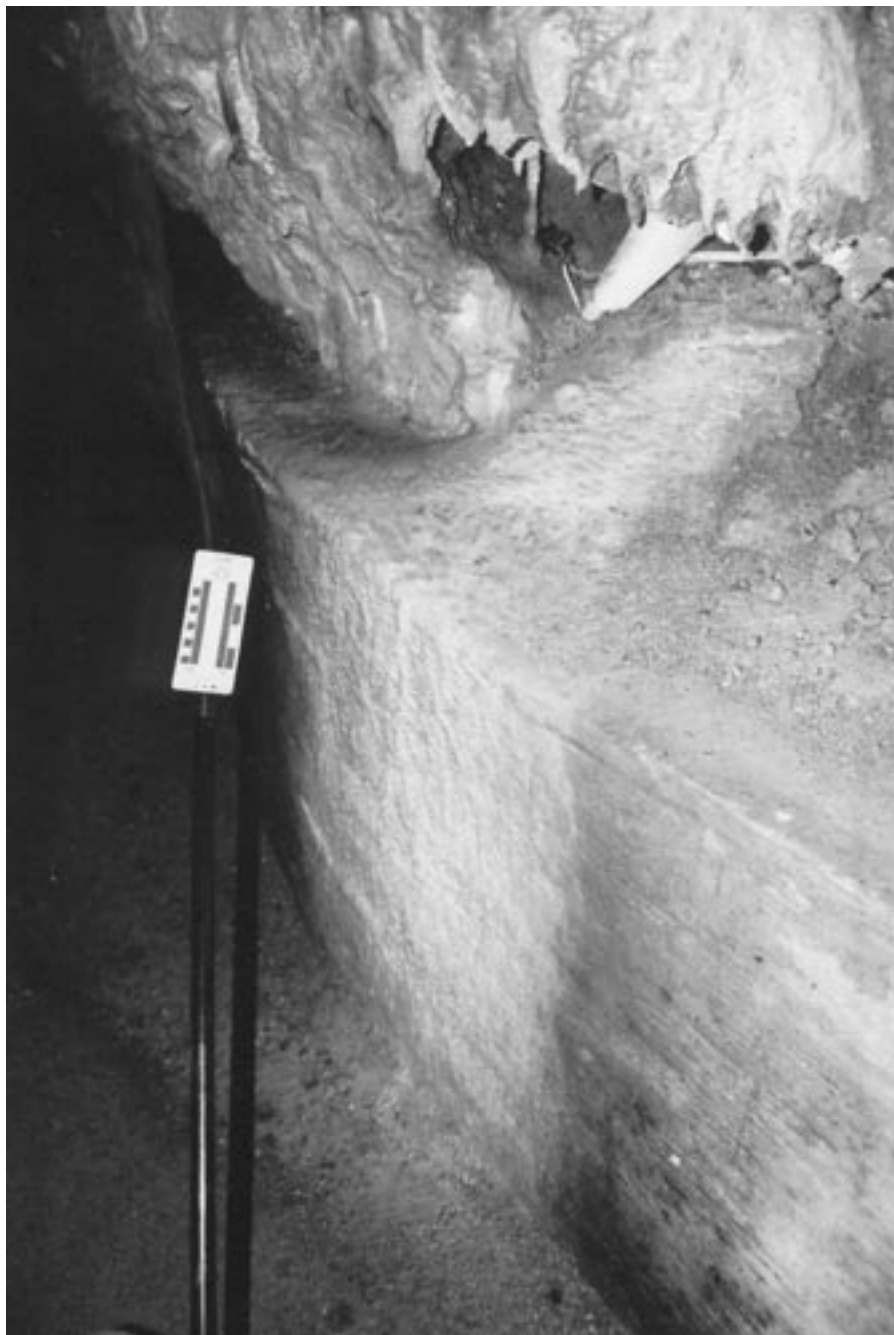
Figure 5. Flowstone is being formed on loose sediment above and to the right of this 40-year-old concrete wall, covering the top of the wall and flowing down its side onto the cave floor. Many small rimstone dams and their pools occupy much of the area of the deposition above the wall and also continue forming on the upper part of the wall. Scale in cm and in.
