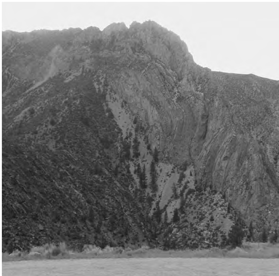
Figure 7. High angle reverse fault in the northeastern Uinta Mountains. Uinta Group quartzite on the left and Paleozoic sedimentary rocks on the right.
