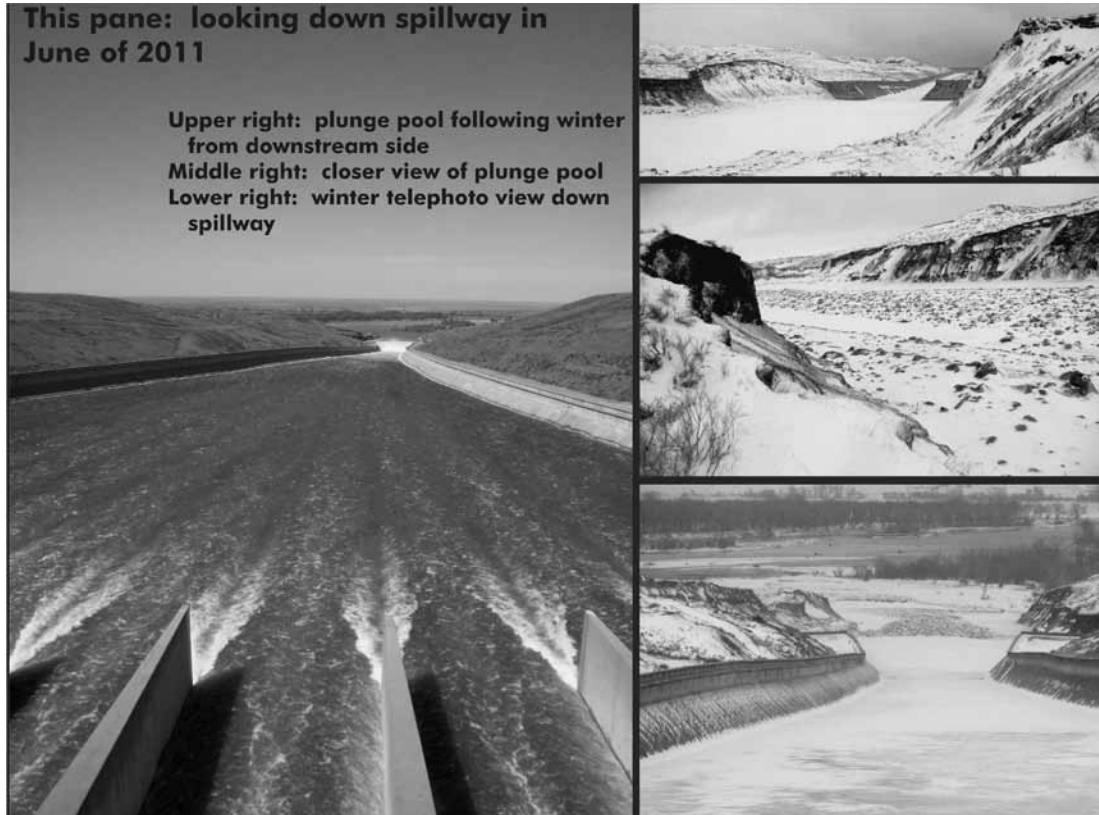
Figure 12. The spillway for Fort Peck Dam is located away from the dam in terrain eroded into Bearpaw Formation sedimentary rocks.
