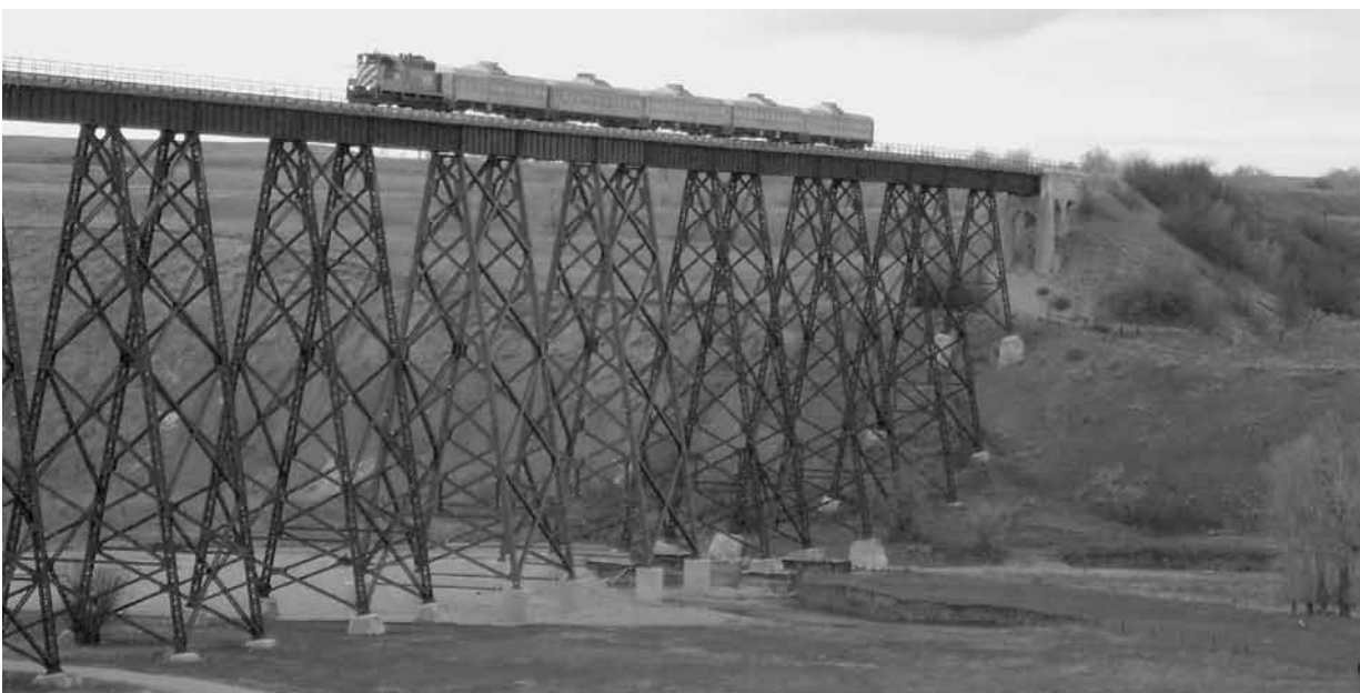
Figure 10. The first revenue train following repair of the viaduct was the Charlie Russell Chew Choo dinner train on November 21, 2014. Grain trains still had to wait for repair of the Ross Fork Bridge. Note the new piers supporting bents directly under the train. Photograph courtesy Central Montana Rail.
