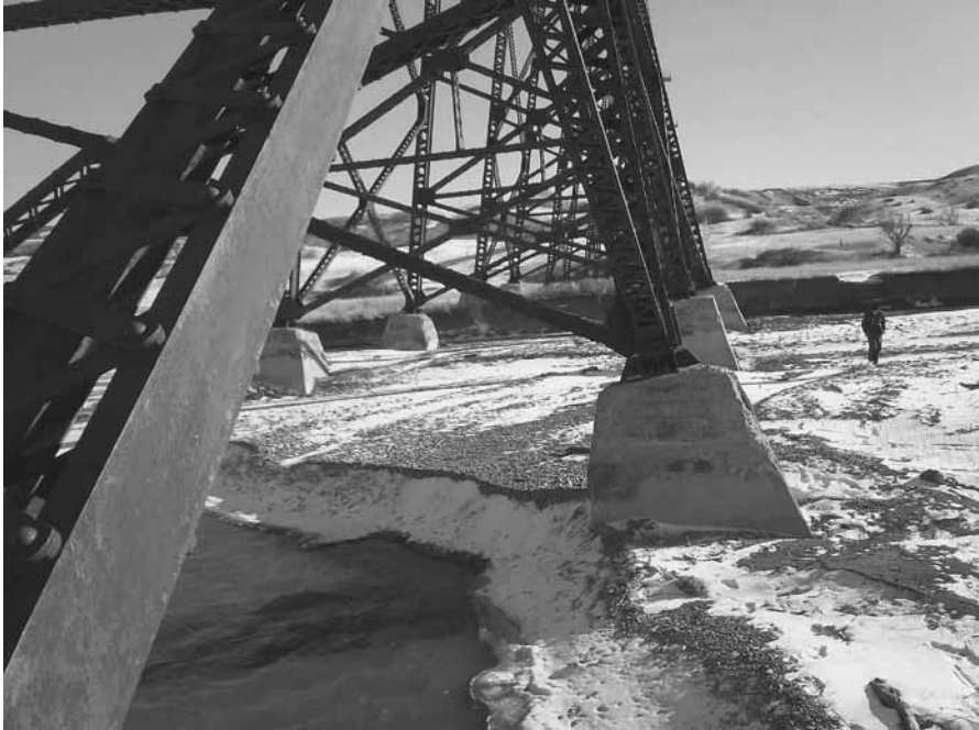
Figure 11. Wide gravel bar deposited by 2011 flood buried the pre-2011 river channel. Author (at right) provides scale.
