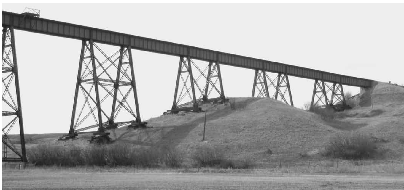
Figure 5. Central Montana Rail trestle over Ross Fork of the Judith River.
