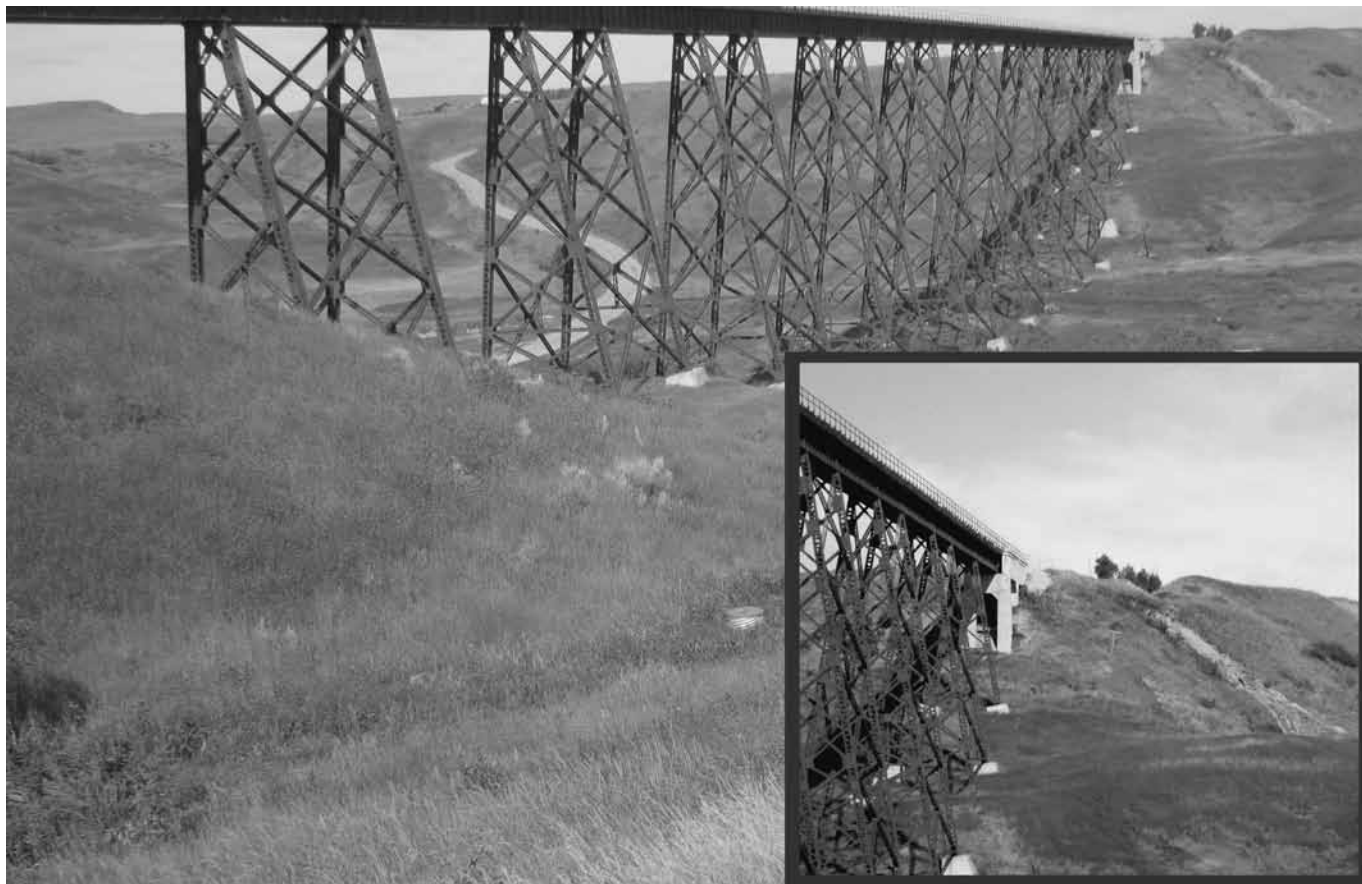
Figure 4. Central Montana Rail bridge over Indian Creek southeast of Danvers, Montana.
