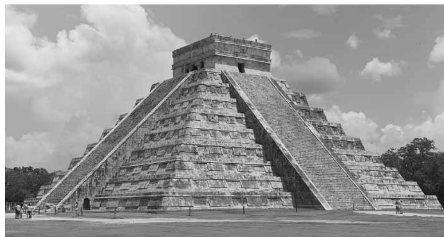
Figure 3. The Temple of Kukulcan (El Castillo) at Chichen Itza in the Yucatan, Mexico (built 600–1000 AD), is typical of a basic ziggurat, also called a stepped pyramid. The basic features are the layers of receding steps, with one or more stairways, and a shrine on top. Variations of this design are seen around the world. (Wikipedia: Photo by Pedro Marcano, August 2014.)
