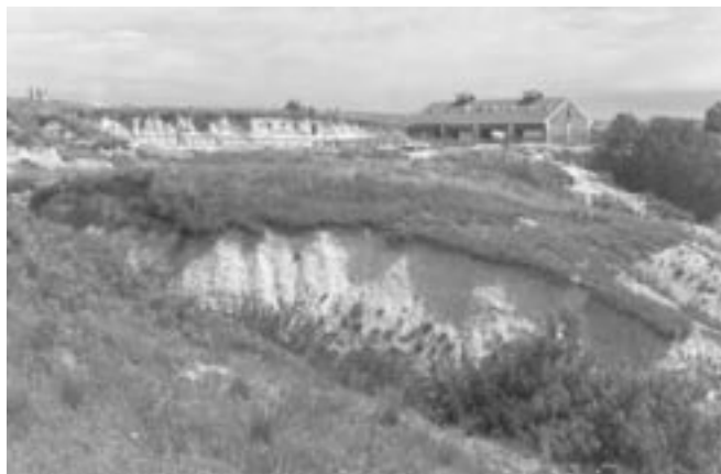
Figure 2. The Rhino Barn houses the megafossils that have been excavated and left in situ. Adjacent to the building is a ravine (shown in the lower part of the photograph) carved by headward erosion of a tributary of Verdigre Creek.
