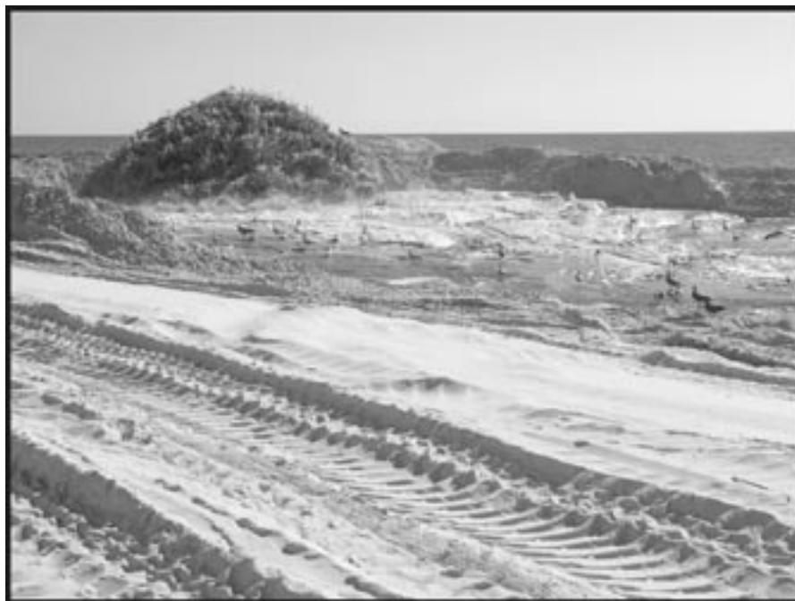
Figure 2. Active beach nourishment along Panama City Beach, Florida. The image is from January 2006, and shows the manner in which the sand-water slurry is pumped onto the beach. The water drains leaving sand deposited under energetic aqueous conditions. The water-sand plume is approximately 8 ft in height.
