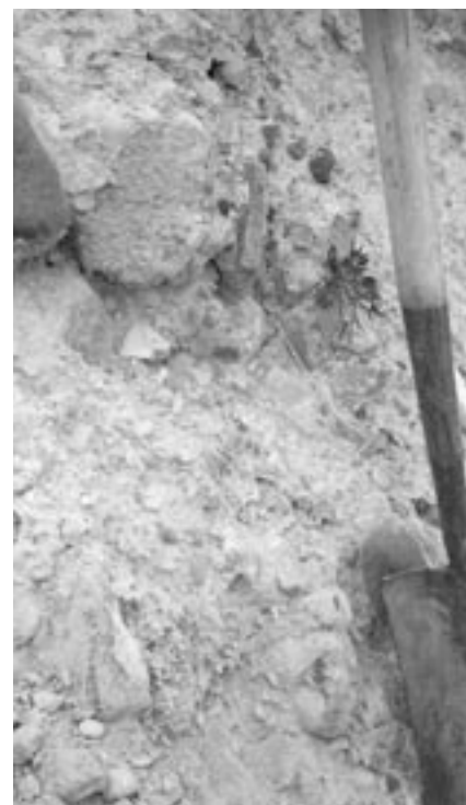
Figure 20. A spade was used to hand excavate in and along previous test trenches (SM-4).
