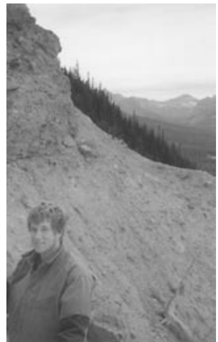
Figure 8. Unstable slope (center scarp), Saint Mary Ridge.
