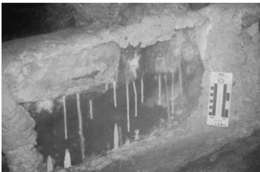
Figure 4. Stalactites, stalagmites, and columns that have formed since 1977 and are still growing. Scale in cm and in.
