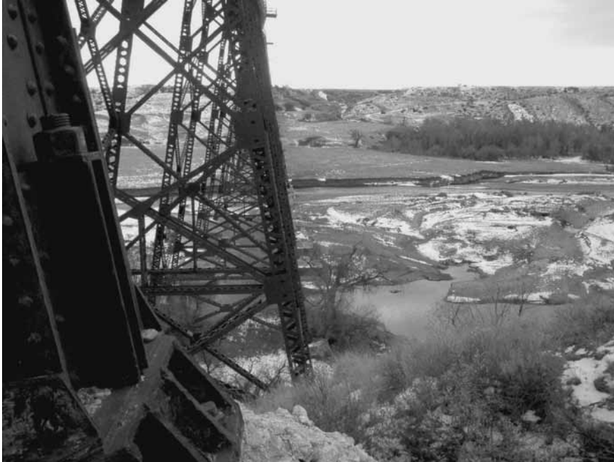
Figure 8. Judith River in Central Montana from west end of Central Montana Rail trestle. Meander migrated down valley (right to left) and abandoned former channel (midground) during 2011 flood. New channel is at east (distal) side of flood plain. Note channel forms in floodplain gravels that might suggest a long period of meander migration with each curved form representing a distinct flood, but this was not the case.
