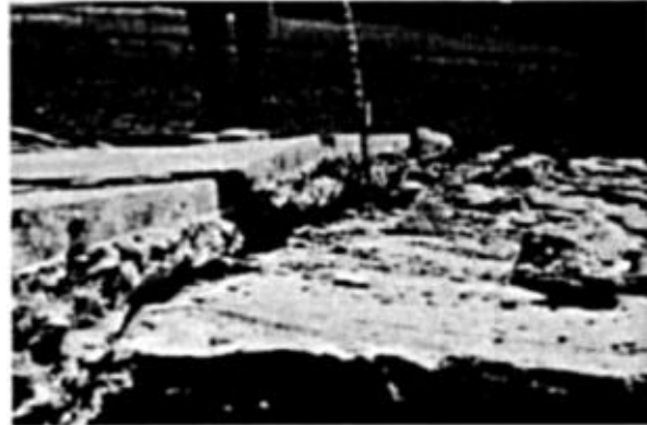
Figure 2. Interstate 210 fault line in concrete: closeup. Here actual overthrusting occurred. Slab to left was elevated more than nine inches higher than that at right and moved across the other slab during the earthquake. This site provides an excellent model of overthrusting. Note the ground concrete and powdered material nearby. There were striae apparent on the surfaces which rubbed against each other.
