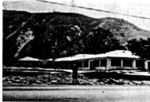
Figure 5. Foothill Boulevard escarpment. Despite road repair, the great vertical component of the San Fernando earthquake is fully evident in this view toward the northeast.
