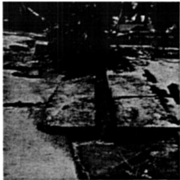
Figure 10. Closeup view of overthrust surfaces, blacktop on concrete. The blacktop slab of Figure 9 was lifted manually and turned so that to the left one can see the surface of blacktop which slid across the concrete to the right. Some sandstone which had been originally beneath the blacktop can be seen as it was moved along with the blacktop. Some evidence of sliding is evident on the blacktop surface but not on the hard concrete. Perhaps a greater weight of sediments atop the blacktop would have caused greater evidence for overthrust action here. Overthrust evidences are not as obvious at this location as they were at the Interstate 210 escarpment where concrete overrode concrete.
