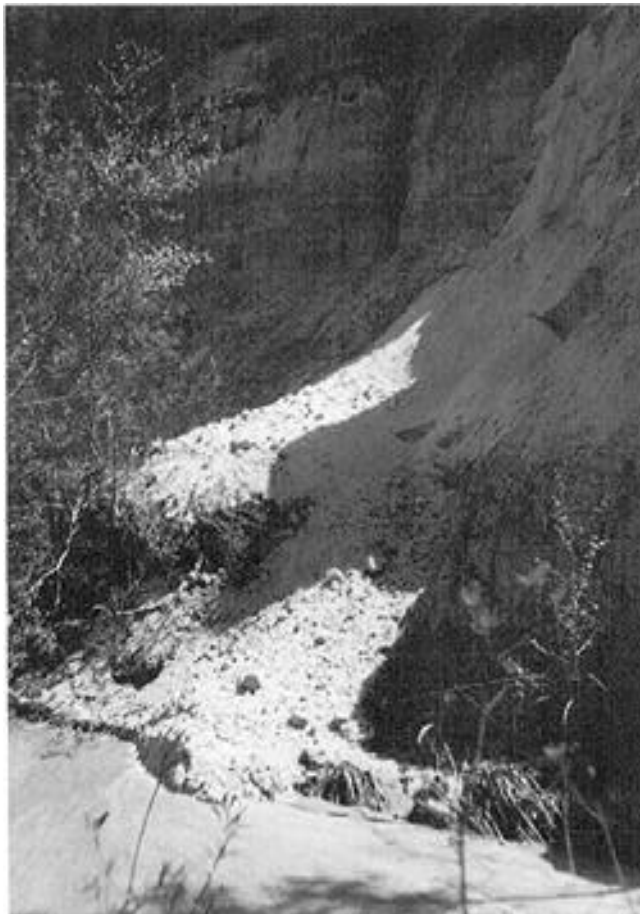
Figure 21. Small alluvial fan formed on canyon floor during the March 1990 cloudburst.
