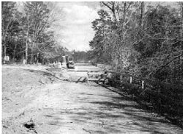
Figure 25. Construction to reroute Park road to avoid continually eroding canyon (1994).
