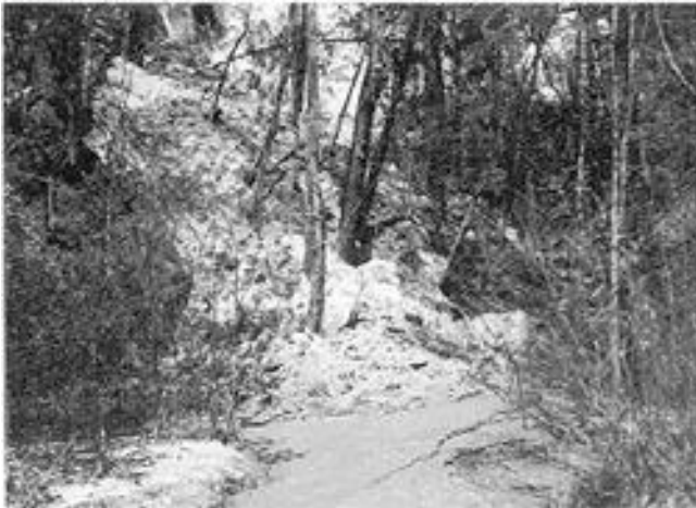
Figure 20. Debris slide containing slump blocks and smaller sections of sedimentary material from freshly-eroded canyon wall (1990).
