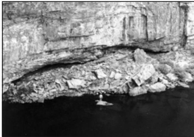
Figure 7. Undercut areas of DeSoto Falls' catchment basin at the elevation of plunge pool. Note talus dike now protecting undercut areas from significant erosion. Person on rock in water provides scale.
