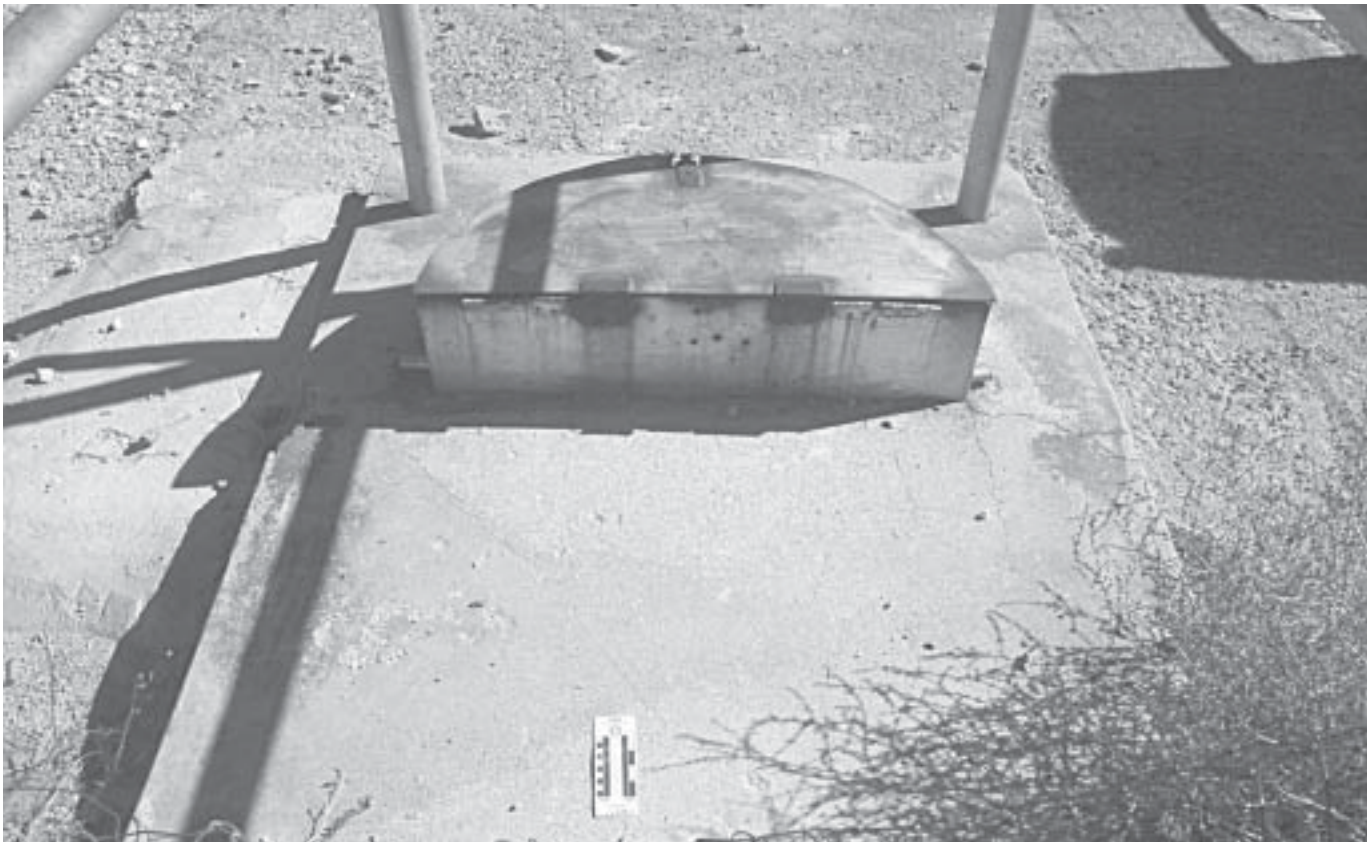
Figure 3. Photograph of the metal cover over the 165 foot-deep shaft also constructed by Sellards and Evans to understand the depth of meteor penetration. Scale in inches and centimeters.
